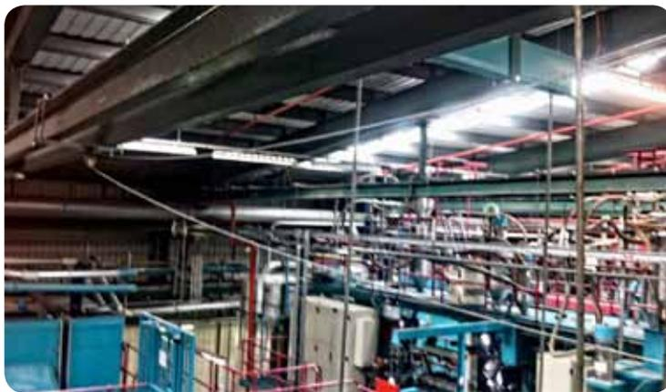
*Each system was easily installed utilising the T-Line's brackets. No intermediate supports were required and the system was ready for use within a few hours.*
