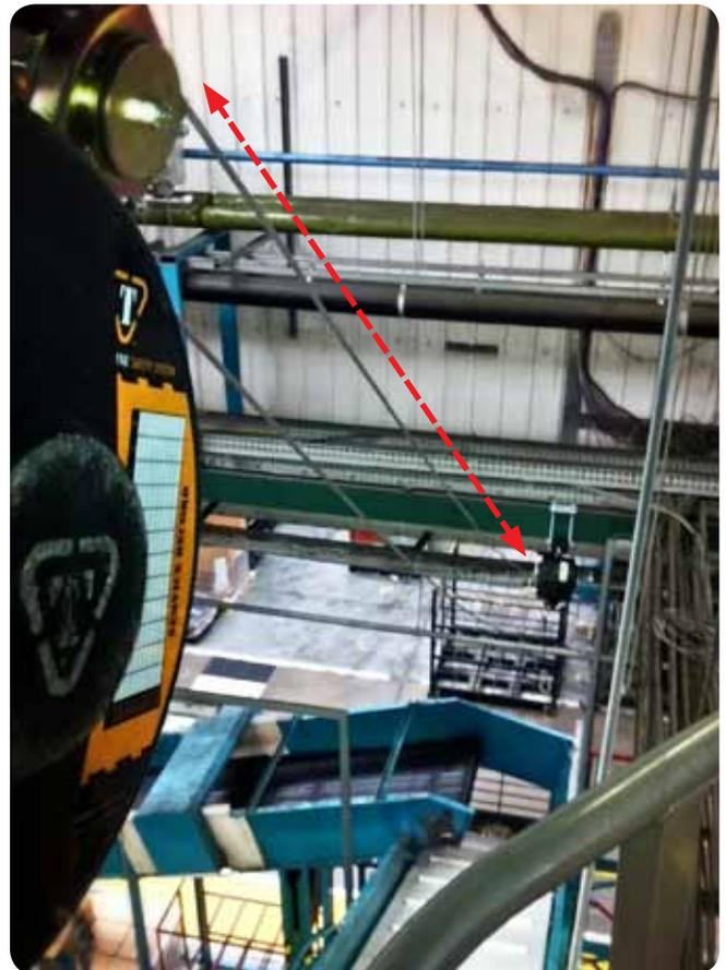
*T-Line mounted above a conveyor, with each end at different heights*
